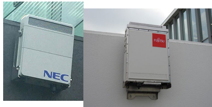
Fig. 9-3 Appearance of millimeter wave RU (by NEC, Fujitsu)
